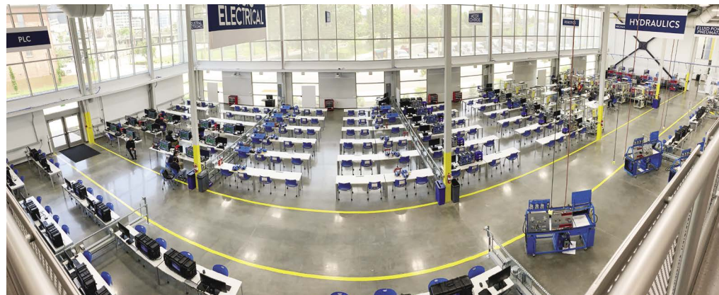
A bird’s eye view of the Louisville FAME Technical Center. (Provided by The Manufacturing Institute | National Association of Manufacturers)
